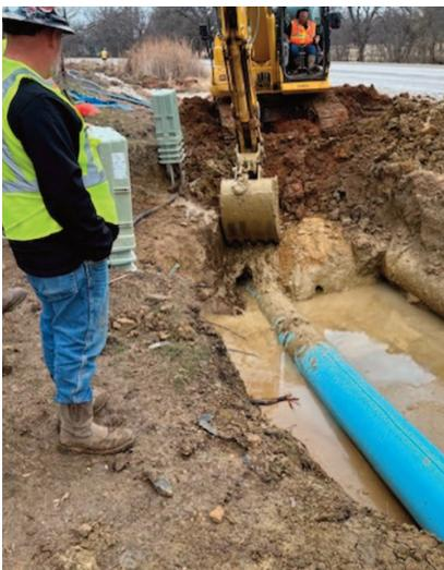
Figure 5. Boring pit showing a high groundwater level
