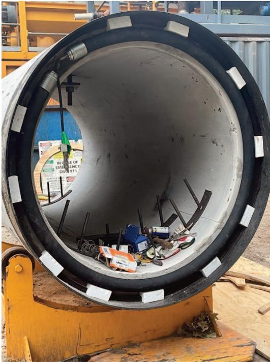
Figure 5. RCP hydraulic joint configuration
