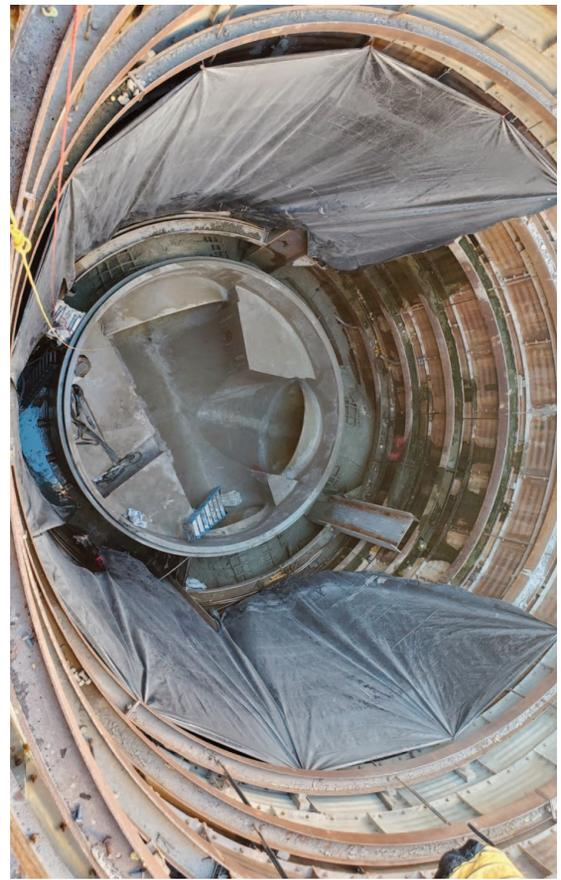
Figures 6 & 7. Polymer Concrete Structure Field Assembly
