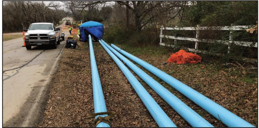
**Joint fusing and pipe staging area. Sticks of PVC are joined to full run length prior to the day of the burst, stored conveniently out of the way near the insertion point**
