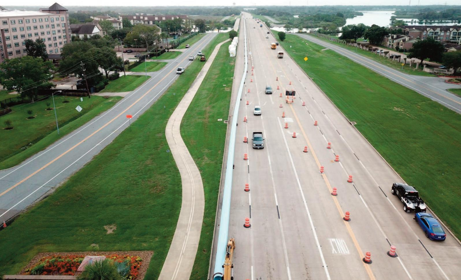
**Figure 4: HDD Pipe Staging along Egret Bay Blvd.**
