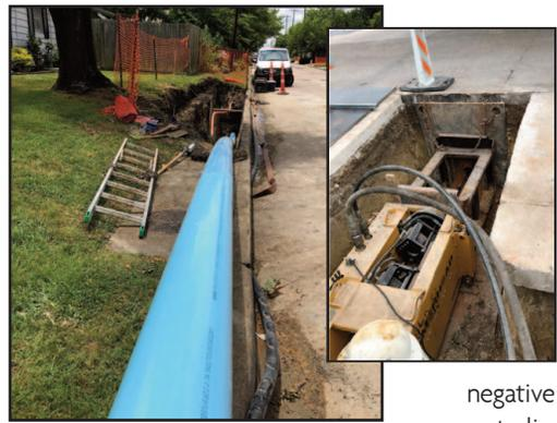
**Minimal excavation/restoration.** The pipe bursting method reduces digging requirements are reduced as much as 90 percent compared to an open cut "dig and replace" method. The only excavation required is for the pulling machine, insertion pit and accesses to service connections
