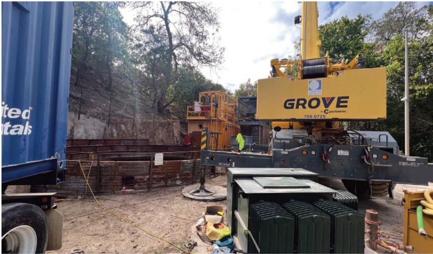
Figure 7. Site constraints limited launch and receiving pit locations
