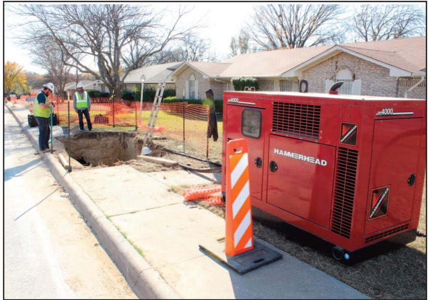
*Machine pit dimensions need to be only big enough to accommodate a 4-foot by 12-foot shore box, at a depth not much deeper than the lay of pipe being replaced*
