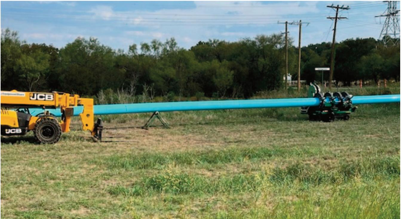
Figure 4. 20-inch fusible PVC pipe
