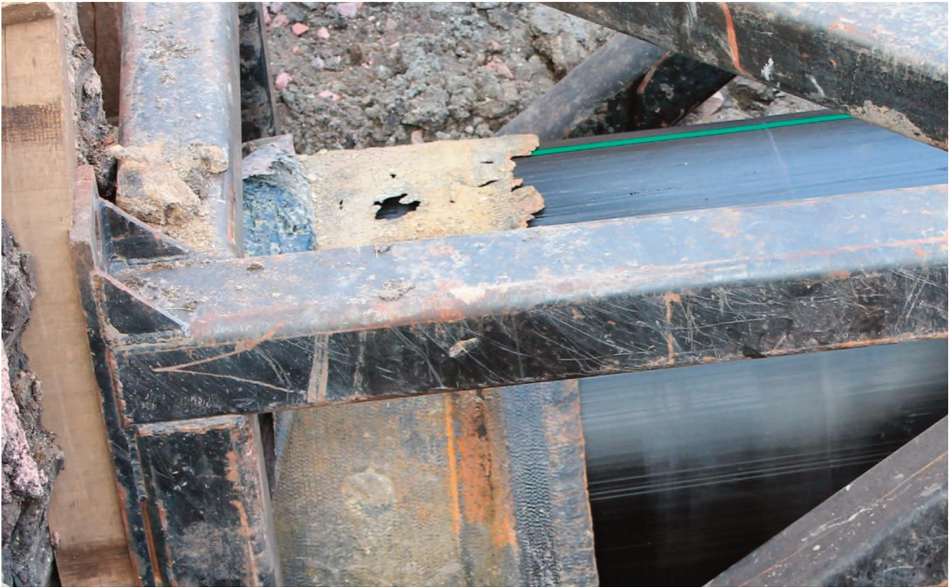
Replacing the corroded ductile iron pipe that had been eaten away by sulfuric acid caused by sewage, the HDPE pipe is inserted into the destroyed pipe using the CompressionFit method from Murphy Pipeline (Photo credit: Murphy Pipeline)
