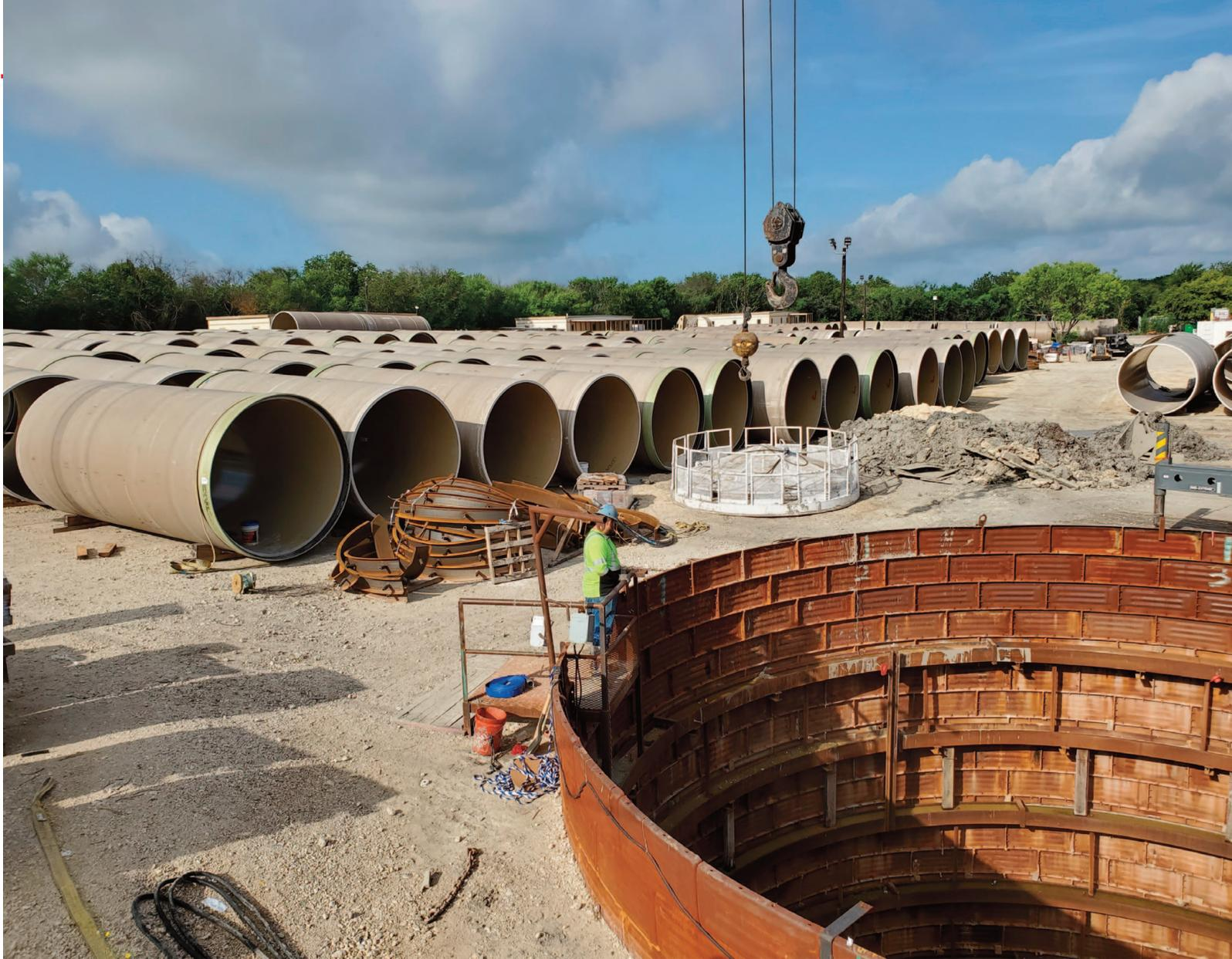
**Figure 5. Hotel Shaft Site and FRP Pipe Ready to be Installed**
