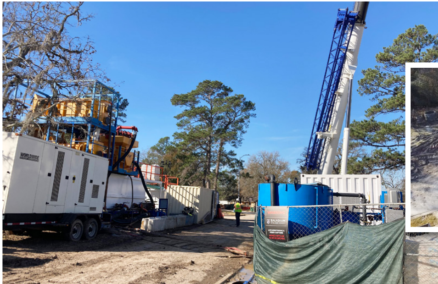
Microtunneling equipment set-up at jacking shaft MH-T12 on Talton St.
