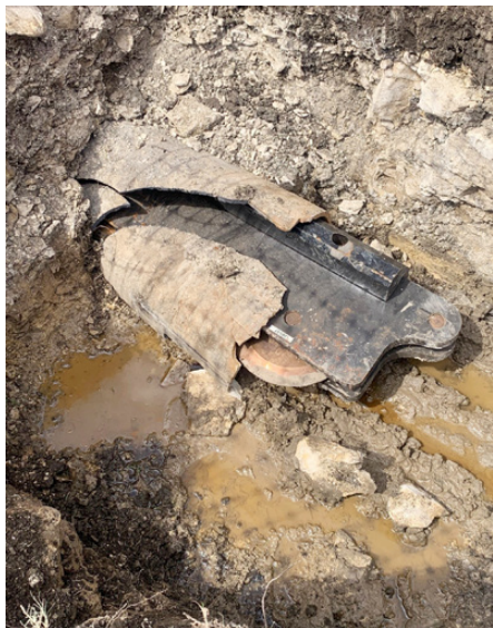
Static Pipe Bursting Head / Cutter
