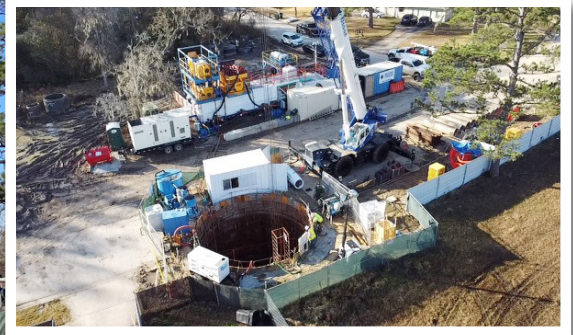
Microtunneling equipment set-up at jacking shaft MH-T12 on Talton St.
