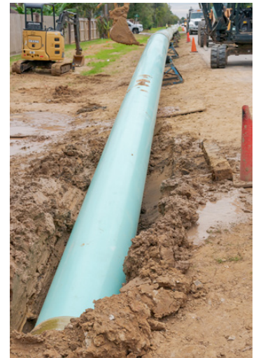
HDD is an efficient installation method in congested, primarily residential, rights-of-way
