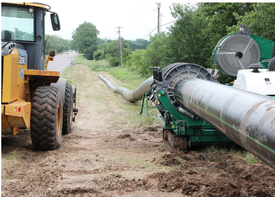
Ability to fuse several hundred feet means quicker installation
