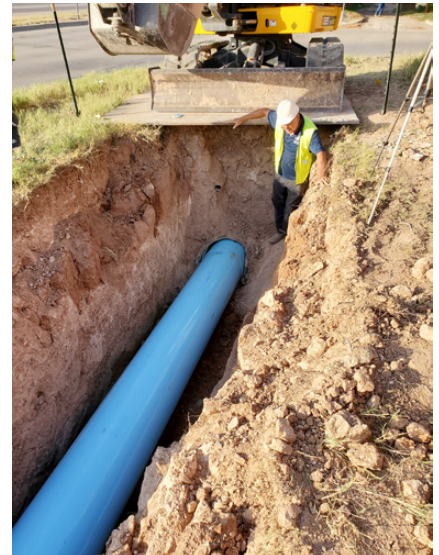
Over 99 percent of the line was installed via standard sliplining
