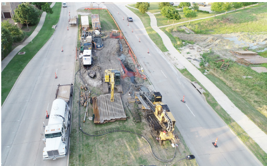
Figure 4 - HDD Entry Pit and Staging Area
