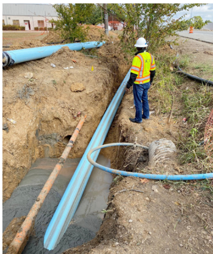
Horizontal Directional Drilling of Fusible PVC® Pipe
