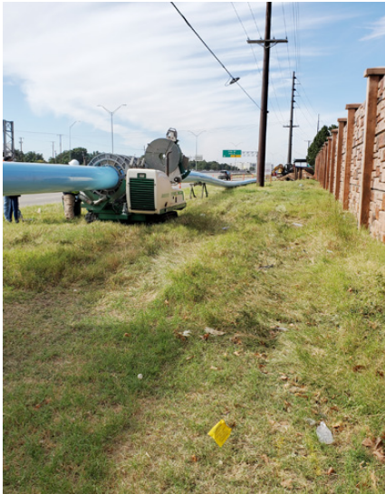
Due to the congested ROW, a trenchless rehabilitation method was selected
