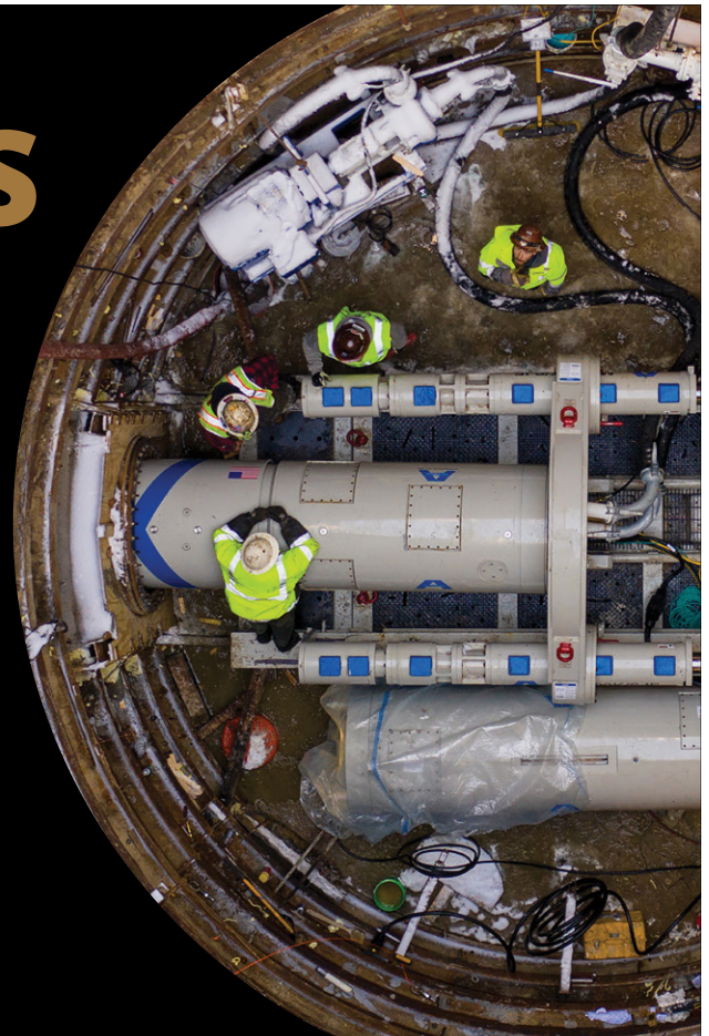
Massive scale of the wet well and pumps required a crane
