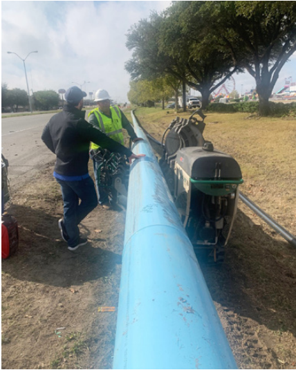
Fusible PVC® Pipe Being Fused
