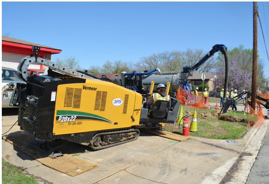
Drill rigs work side-by-side with the vac trucks
