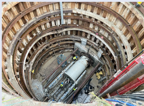
Flowing ground and high hydrostatic pressure created challenges during shaft construction
