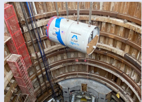
MTBM included a mixed face cutterhead designed for varying ground conditions
