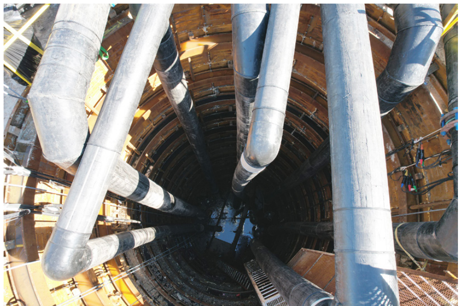
A 65 foot deep shaft was built to house the temporary wet well
