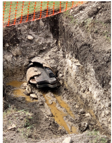
Static Pipe Bursting Head / Cutter
