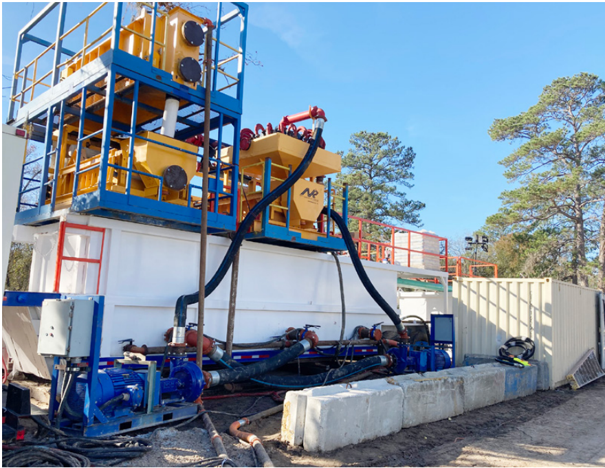
Separation plant set-up at jacking shaft MH-T12 on Talton St.
