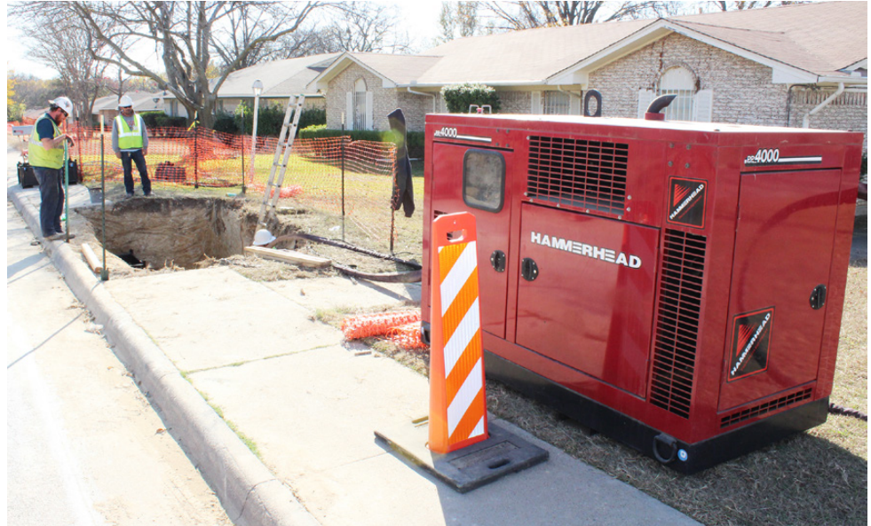
Machine pit dimensions need to be only big enough to accommodate a 4-foot by 12-foot shore box, at a depth not much deeper than the lay of pipe being replaced
