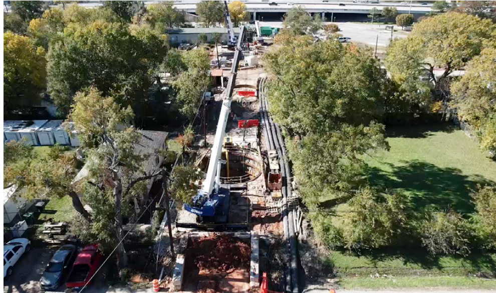
Massive scale of the wet well and pumps required a crane
