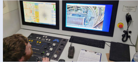
MTBM was remotely controlled and monitored above ground
