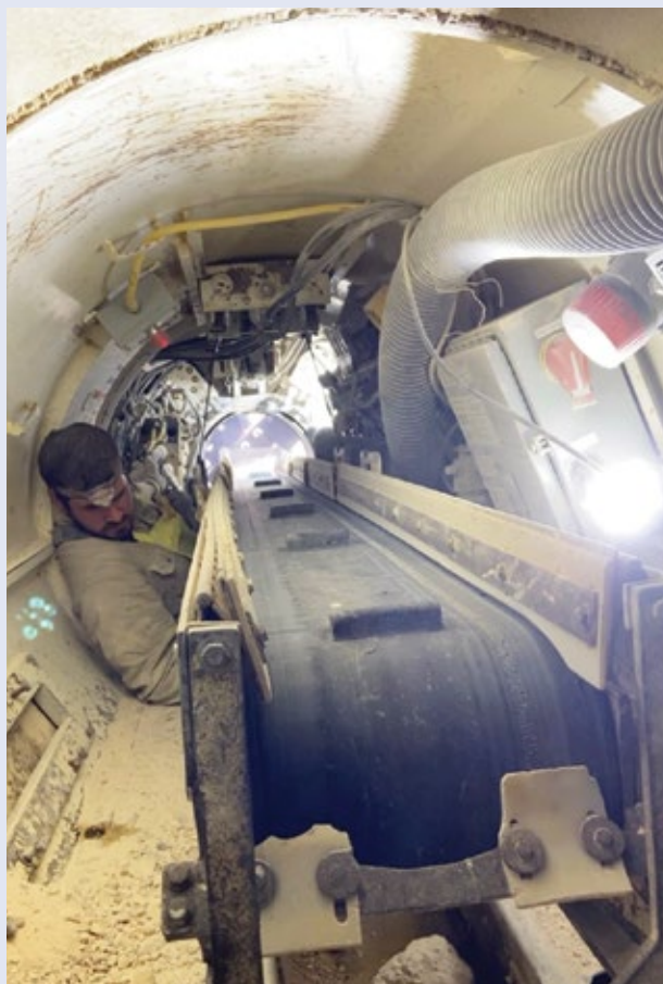
Key benefit of the Akkerman TBM is ability to access the face for obstruction removal
