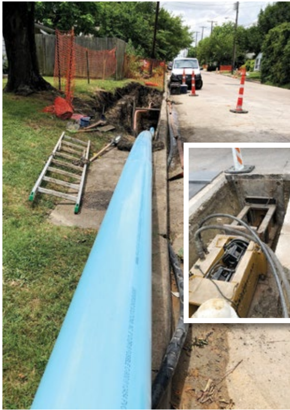
Minimal excavation/restoration. The pipe bursting method reduces digging requirements as reduced as 90 percent compared to an open cut “dig and replace” method. The only excavation required is for the pulling machine, insertion pit and accesses to service connections
