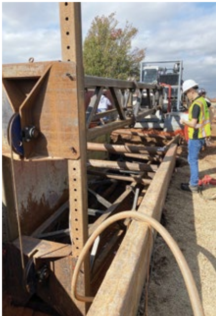
Figure 6: Winch and 90° Pulleys in Liner Receiving Pit
