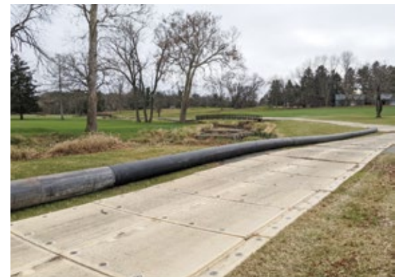
Utilizing matted road for bypass installation reduced damage to the course
