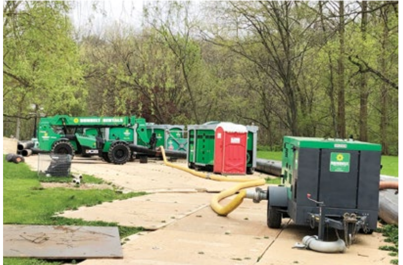
Sunbelt pump solutions team gets started on the bypass
