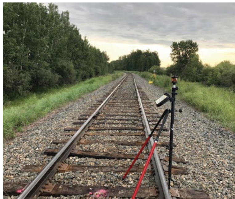
Figure 3: Robotic Total Station or Levels can also be used by qualified personnel to complete the monitoring or construction surveys
