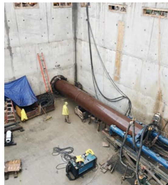
Figure 4. MTBM launch pit from the forebay basin
