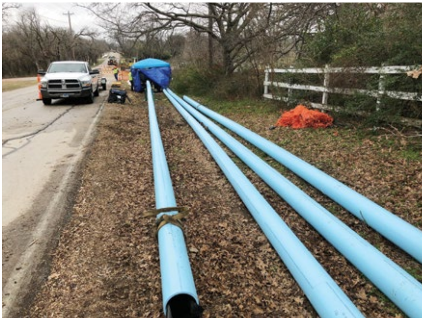
Joint fusing and pipe staging area. Sticks of PVC are joined to full run length prior to the day of the burst, stored conveniently out of the way near the insertion point
