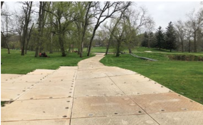
A pinned heavy-duty composite mat road was the best product for this project to reduce damage to the course
