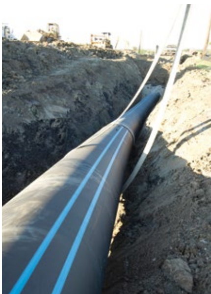
Hydrotesting can be used on runs of HDPE pipe that are hundreds of feet long
