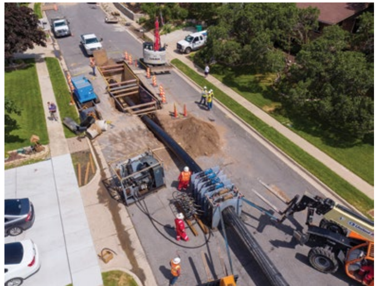
Figure 5: Compressed Fit HDPE Liner Insertion Pit and Roller Box (Aegion, 2019)
