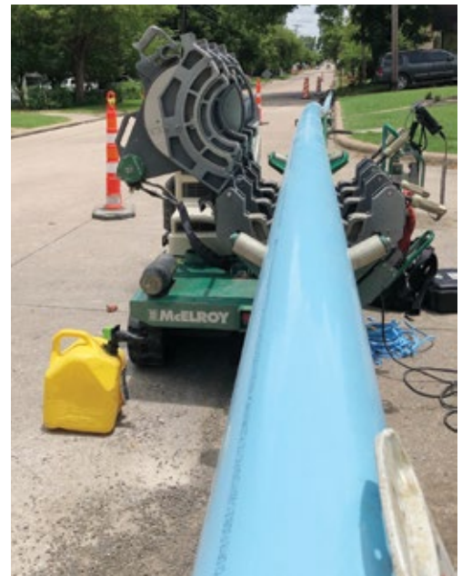
Joint fusing and pipe staging area. Sticks of PVC are joined to full run length prior to the day of the burst, stored conveniently out of the way near the insertion point
