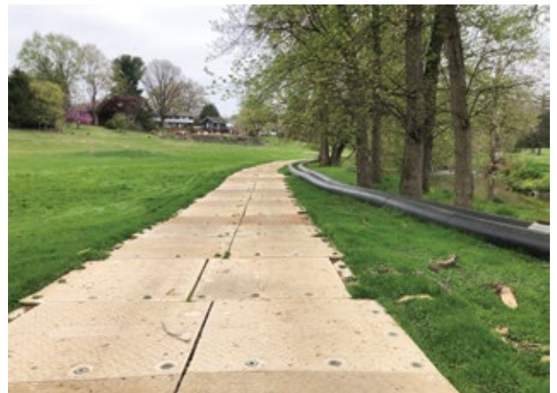
A pinned heavy-duty composite mat road was the best product for this project to reduce damage to the course
