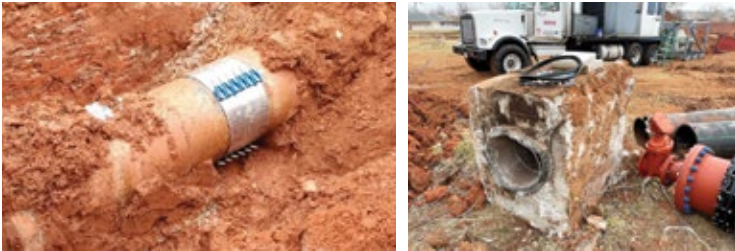
Figure 4: Pipe Repair Collar on Del City Pipeline
