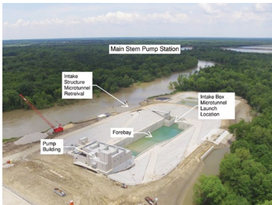
Figure 1. Main Stem Pump Station nearing completion of construction
