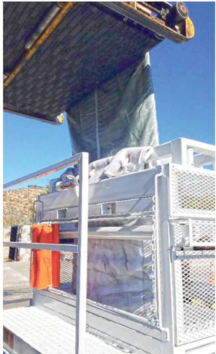
Figure 3 – CIPP insertion
