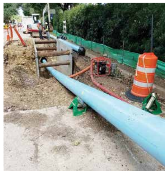
Sliplining using FPVCP supports long pull length and large pull forces
