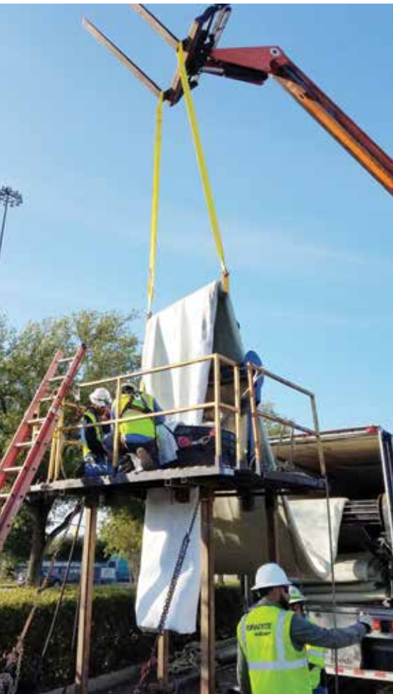
Liners are vacuum-impregnated with a polyester resin
