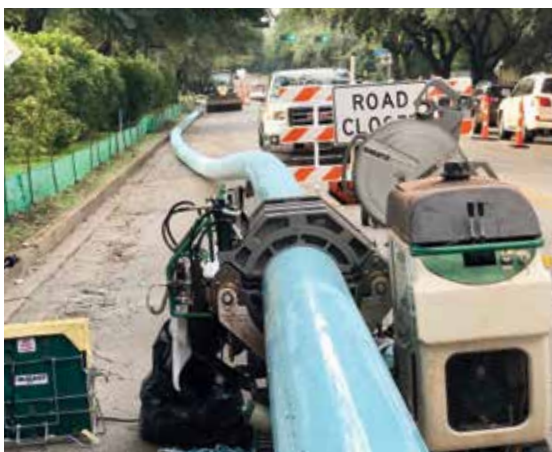
Each joint fusion done was recorded by a data logger on the fusion machine
