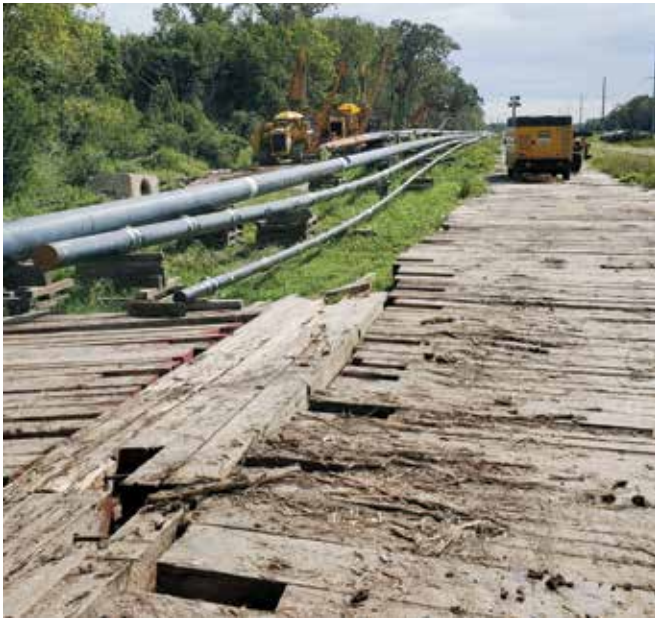
Load-dispersing materials and timber mats placed to protect existing pipelines
