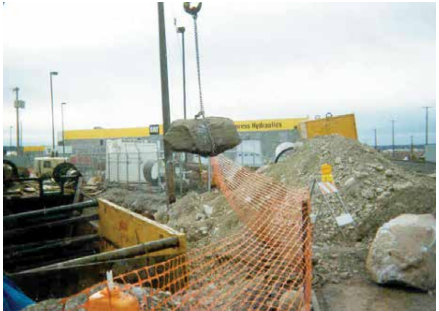
Figure 2- Large boulder removal
