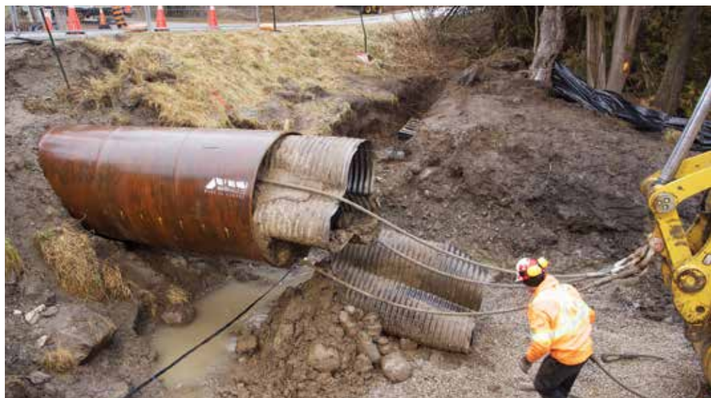
Figure 9- CMP pipe crushing extraction
