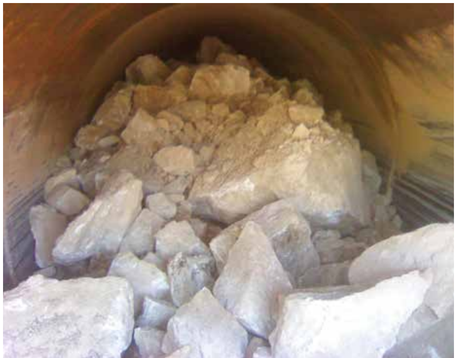
Figure 3 – Spoils inside 60-inch casing
