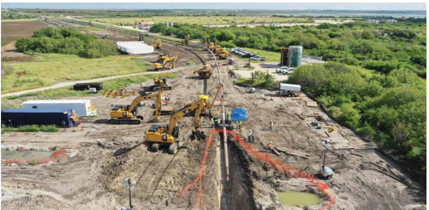
The 9,430 LF of 20-inch steel pipe was welded into one continuous pull string
