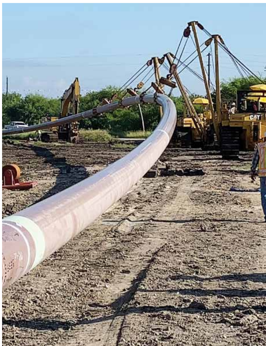
Pipe support is critical to maintain the angles needed for a successful installation
