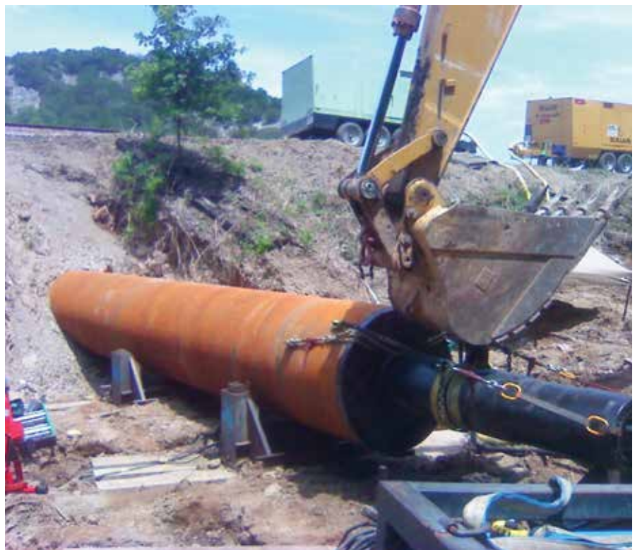
Figure 5- 60-inch casing installation with air compressors sitting on railroad tracks
