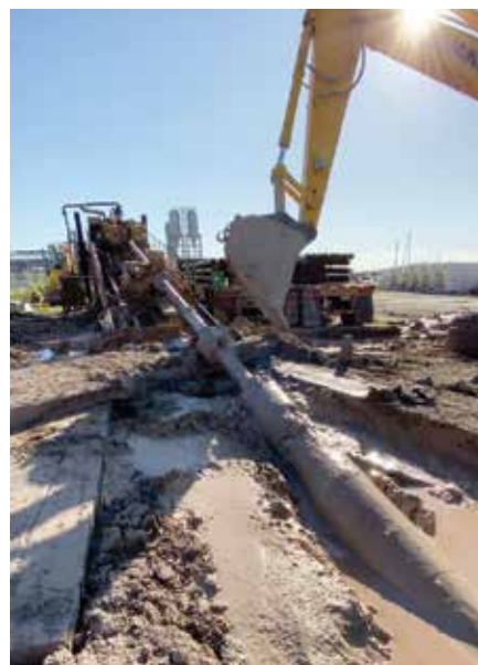
Pulling pressures averaged 450,000 ft/lbs throughout installation with 16 hours total pulling time
