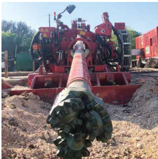
Pilot hole was highest risk part of construction due to potential of intersecting an existing pipeline
