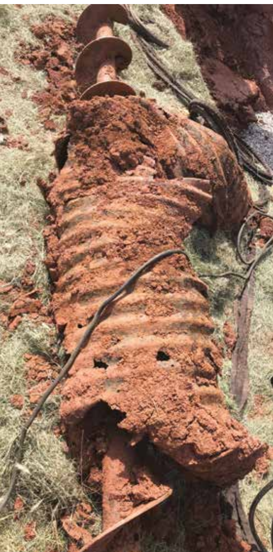
Figure 8- Auger removing CMP in sections
