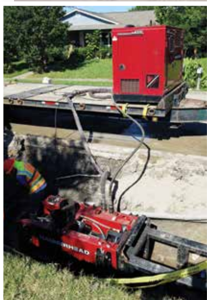
Pipe bursting equipment has compact footprint. Installation was completed and service restored to residents on the same day
