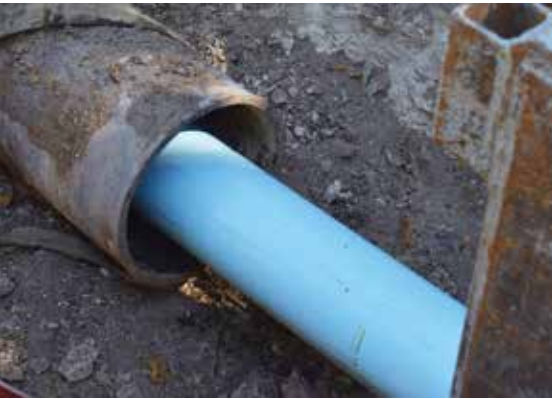
Existing 24-inch main provided suitable casing host pipe for the 12-inch FPVCP
