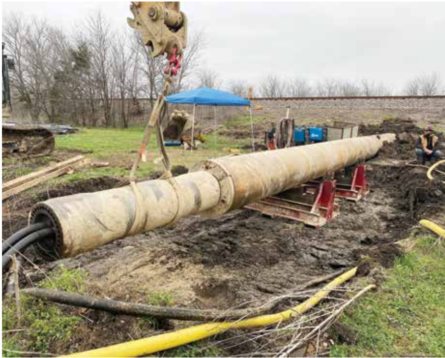
Figure 6- 36-inch casing installation using hydraulic lifting jacks: “Pipe Mules”
