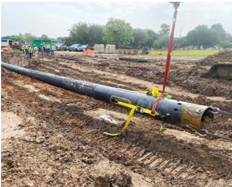
Figure 7- 24-inch Extraction Cradle with 20-inch Hammer replacing 24-inch Pipeline
