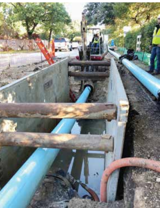
Sliplining method allowed for minimum disruption to existing utilities
