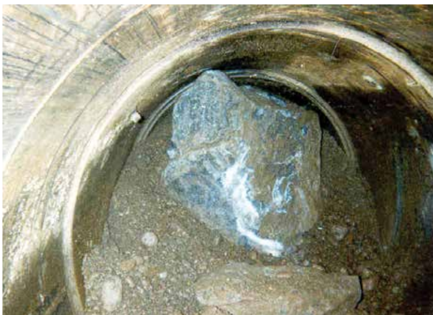
Figure 1 – Boulders and cobble spoils inside casing
