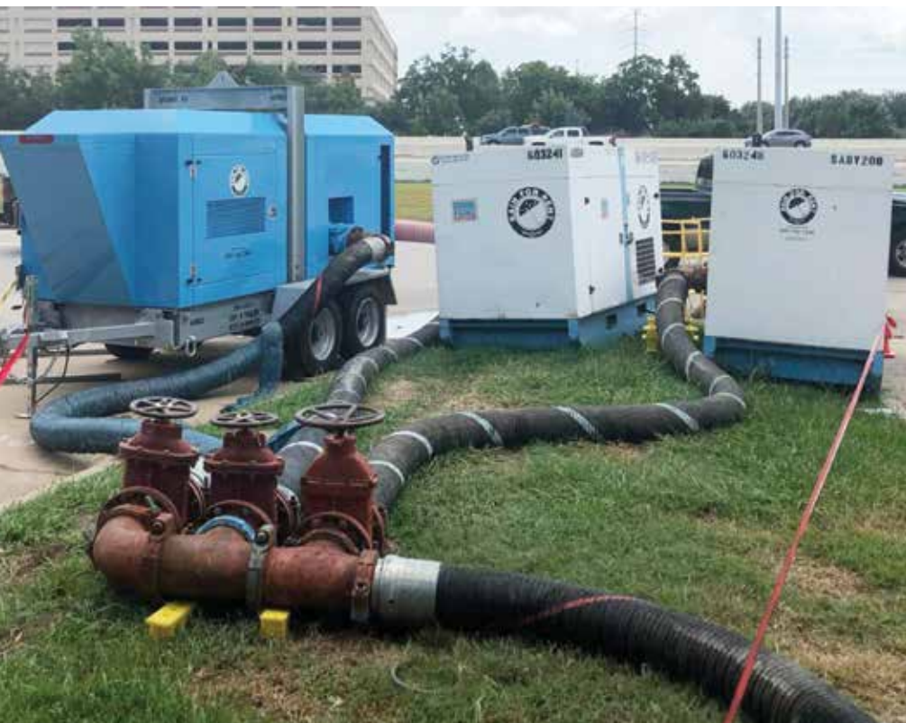
Two-phase bypass for influent lines connected to municipal WWTP. Precise placement of equipment was critical
