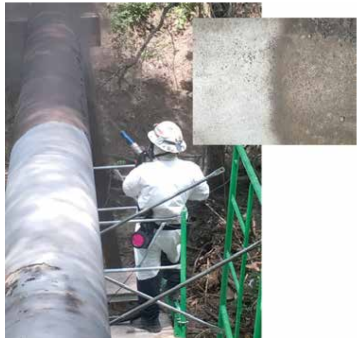
Figure 6: Surface Preparation of Host Pipe
