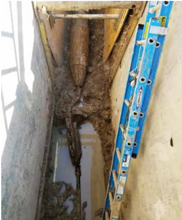
The pipe-slitting operation commences in the entry pit. The string consists of pulling rod, slitting tool and expander connected through flexible linkage, and the new, 12-inch-diameter, HPDE product pipe
