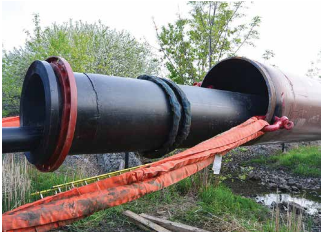
42-Inch Steel Pipe with 24-inch HDPE Ballast Pipe and 6-inch HDPE Fill Line
