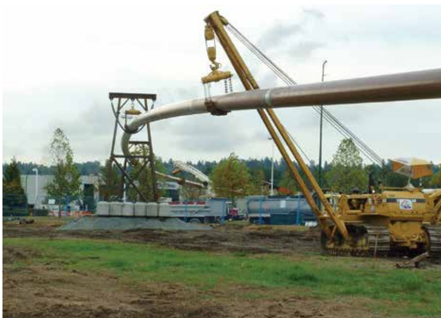
Both vertical and horizontal loads on pipe must be evaluated
