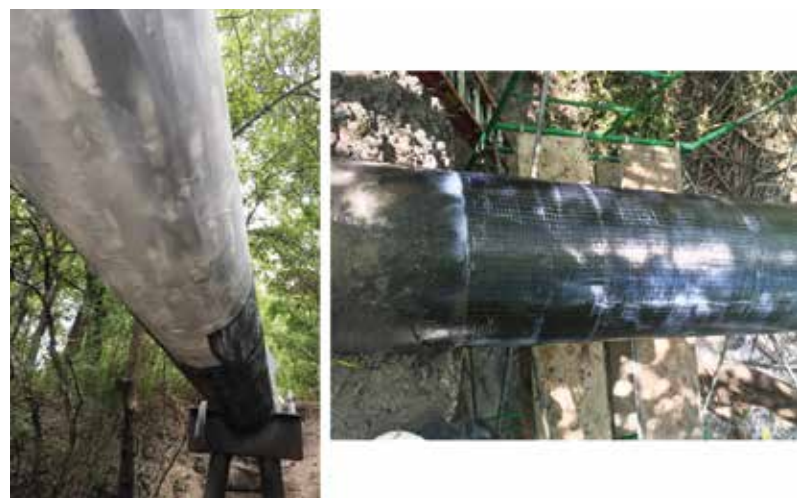
Figure 7: Installation of CFRP System
