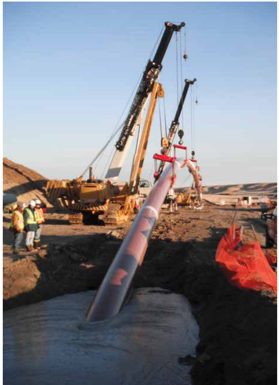
Proper alignment with the drilled hole is critical for safe installation
