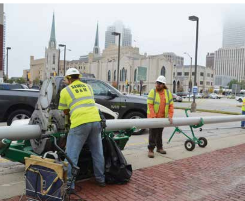
337 LF of seamlessly fused 8-inch HDPE was pulled into place to complete the repair
