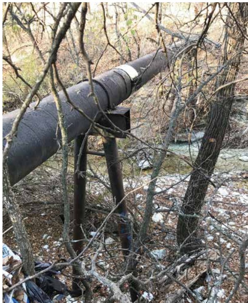
Figure 1. Example of Aerial Pipe to be Rehabbed
