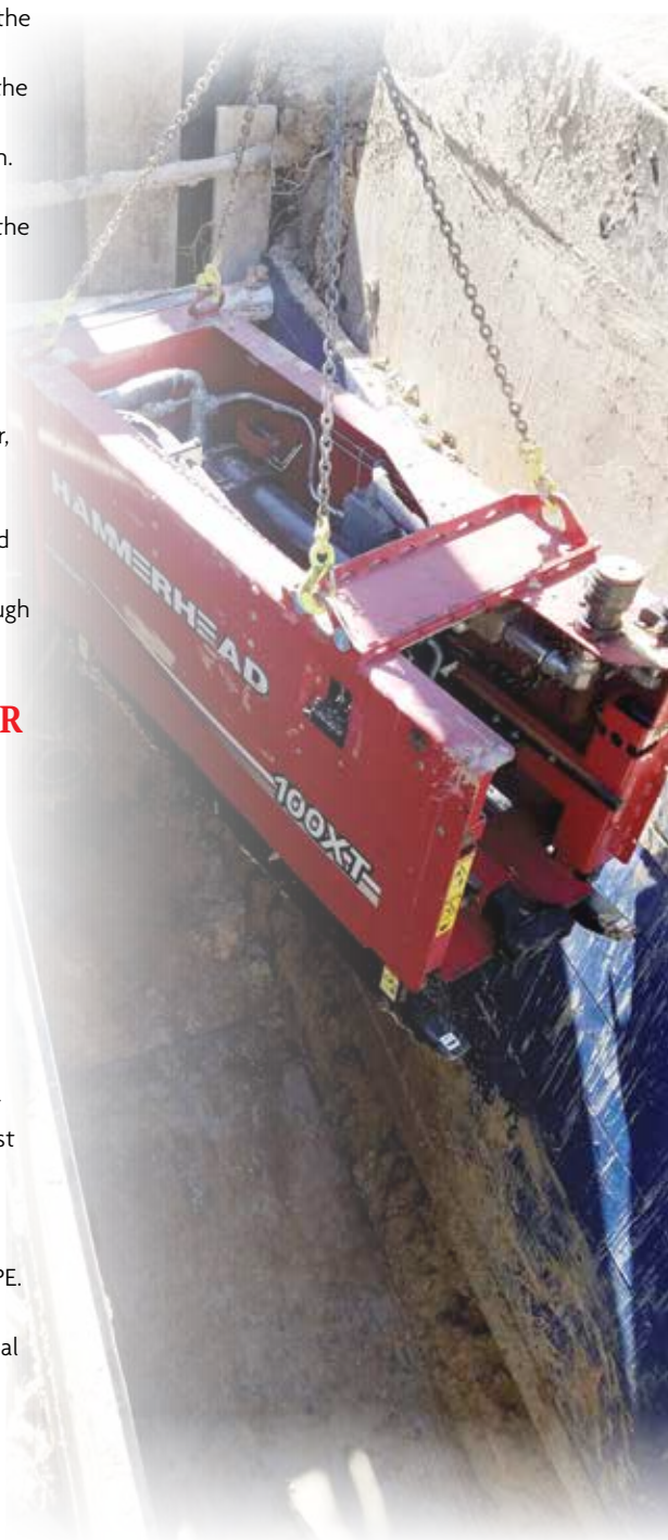
The HammerHead 100XT requires a relatively small machine pit yet has a 100-ton pulling capacity. This pull required 40 to 50 tons psi of pressure through ductile iron
