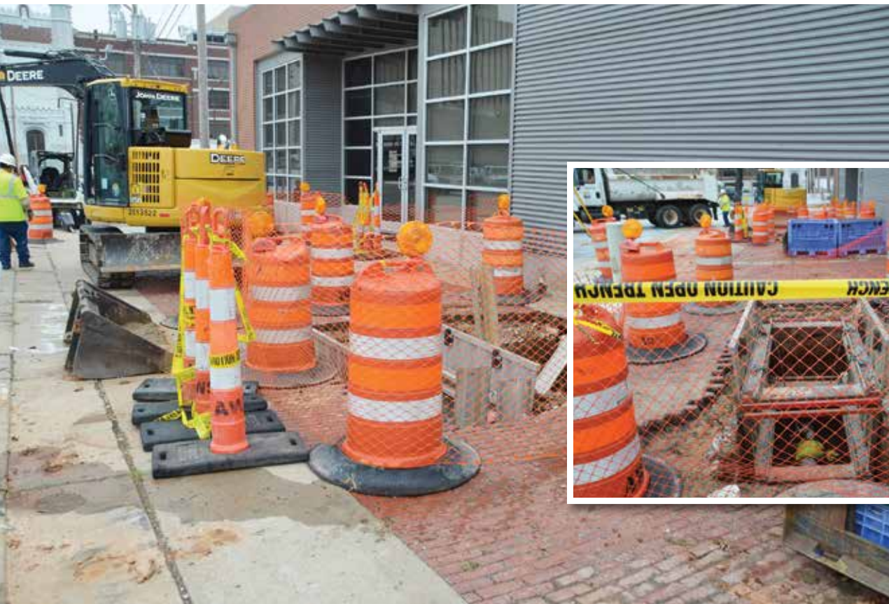
Rented and in-house trenchless equipment allowed City to repair sinkhole without tearing up the street
