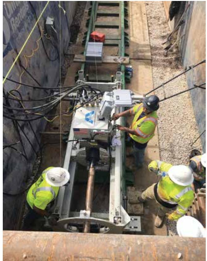
The crew sets up their guided boring and guidance systems to install pilot tubes on line and grade to establish an accurate path for the steel casing
