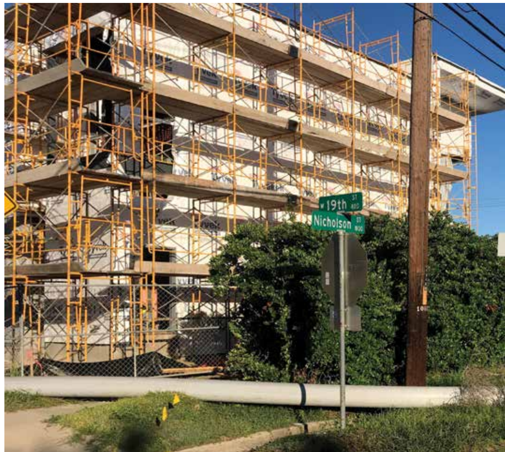
Congested work area permits only one location to lay out fused-up pipe on the surface. It meant pulling through 150 feet of 10-inch ductile iron pipe first from the truss pipe side of a 370-foot run
