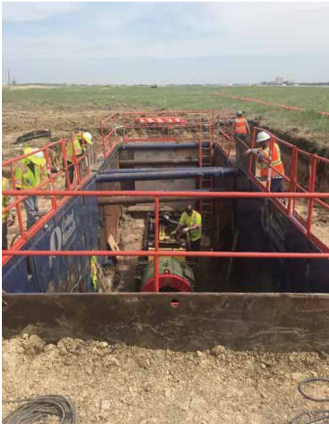
BorTunCo advances steel casing which houses electrical conduit under DFW taxiways that connect to the newly renovated 17C-35C runway
