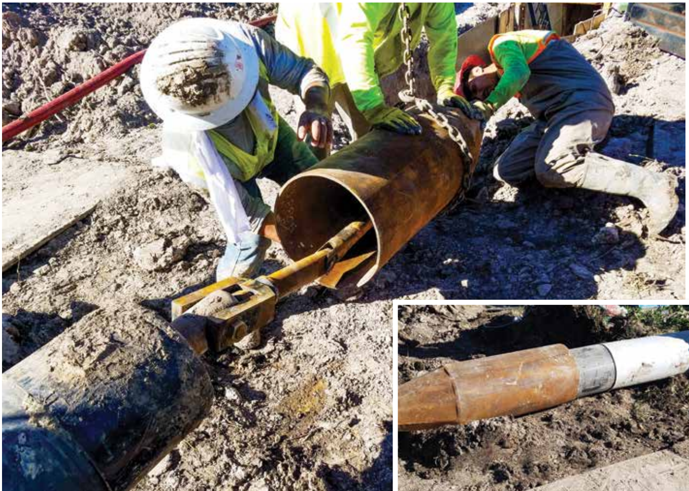
Expander increases the required pipe path by approximately 20 percent of the new pipe diameter, reducing drag for a smoother installation
