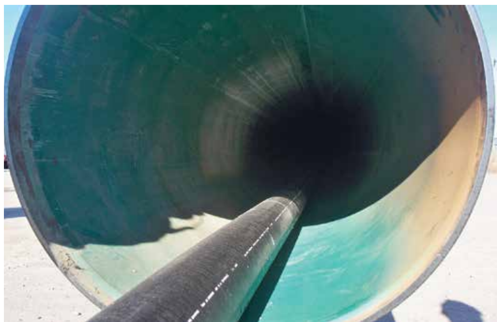
36-Inch Steel Water Main with 6-inch HDPE Fill Line
